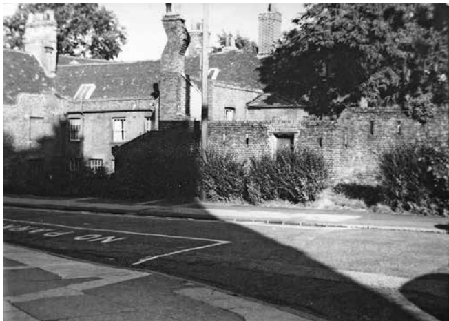
Milton Chantry, initially used for civil defence training, viewed in the later 1950s.
